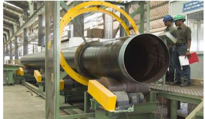
Coating of Pipes
