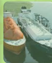
Floating Storage & Regasification Unit (FSRU)
