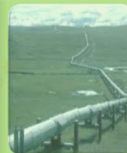
Trans-national Gas Pipelines
