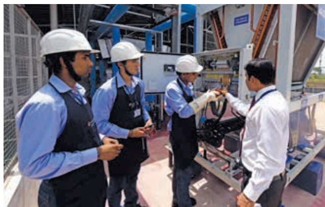
Central air conditioning course at ICICI Academy
