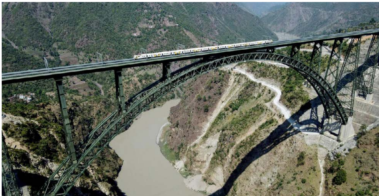
Chenab Bridge High Speed Test Run
