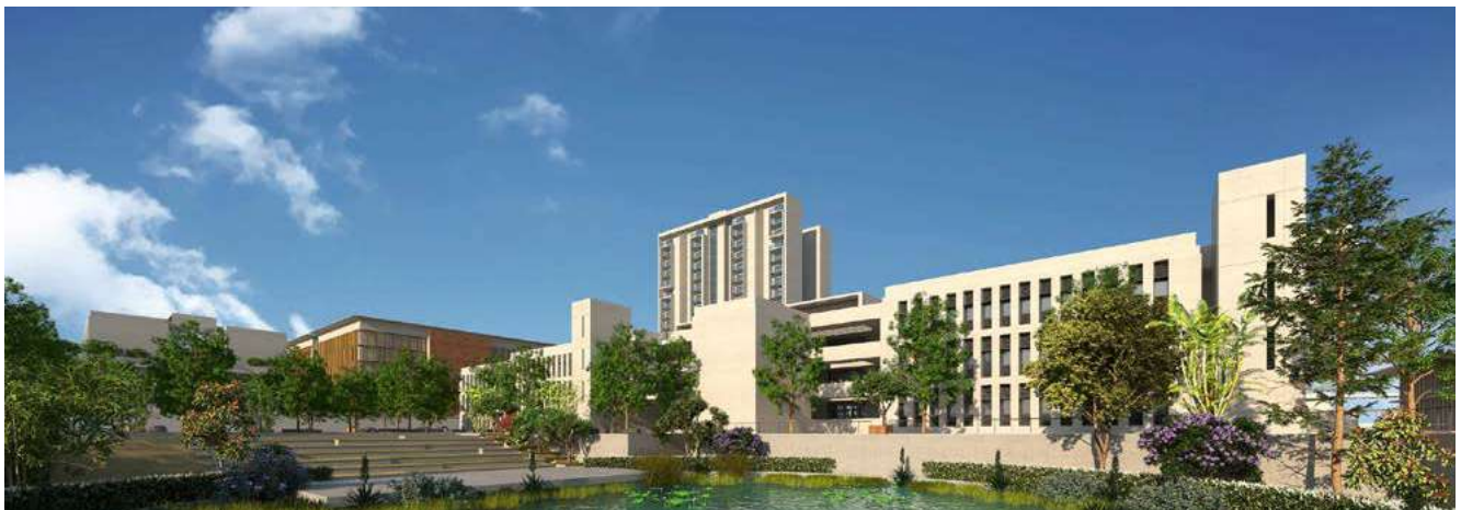
RBI Green Field Data Centre in Bhubaneswar
