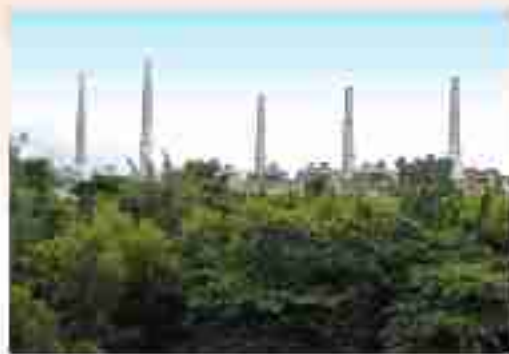
Captive Power Plant
