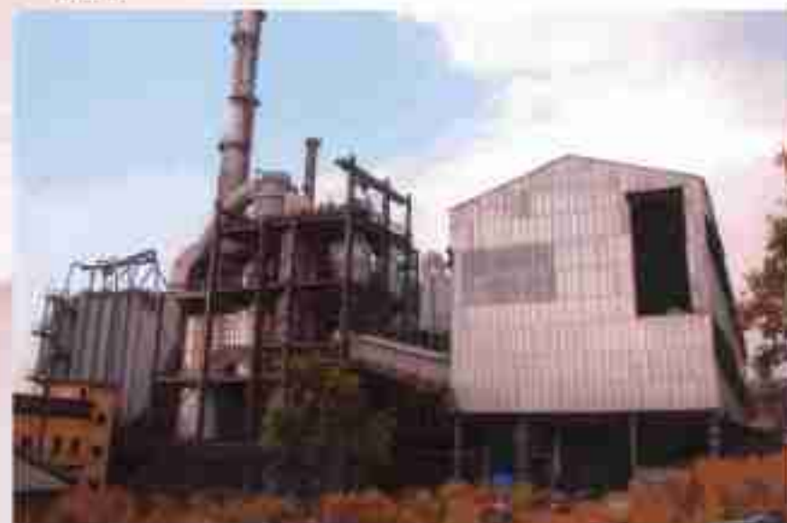
New Calciner Plant at M&R Complex
