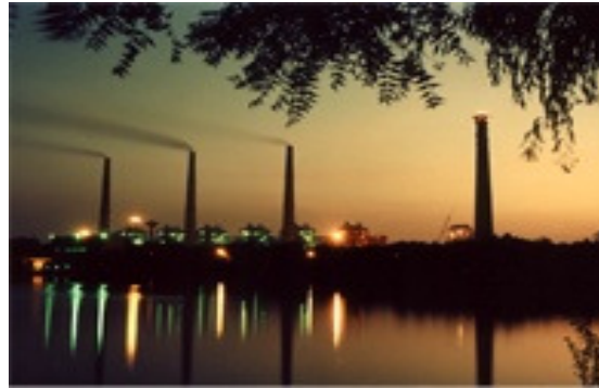
Thermal Power Plant Angul
