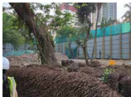
Green cloth covering, site barricading
