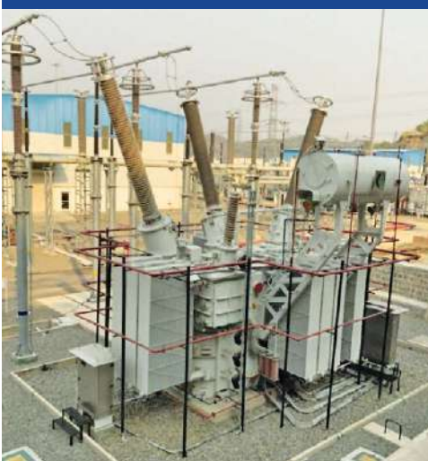
Newly commissioned 125 MVAR, 420 kV Bus Reactor at Kala Amb Substation of PKATL
