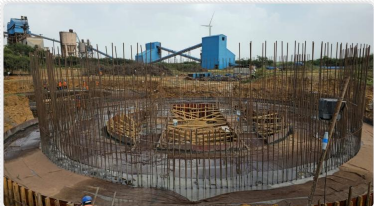
Silo base construction underway at Kutch
