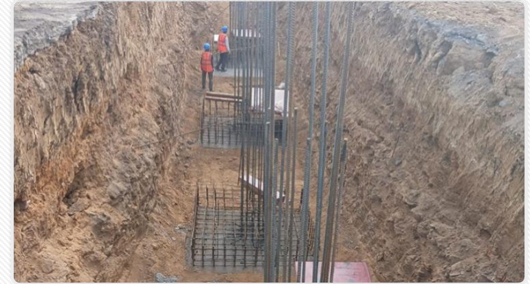
Hopper foundation work in progress at Kutch
