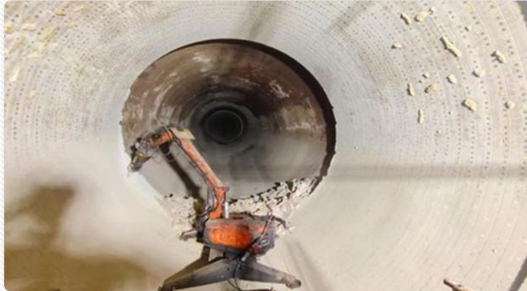
Kiln refractory de-bricking in progress at Kutch
