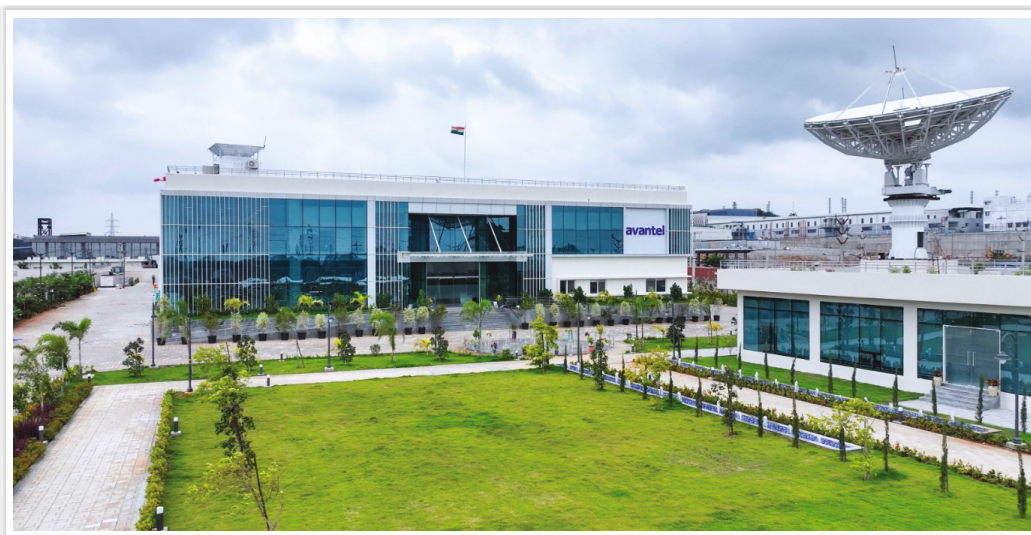
Avantel Limited - E-City Facility, Hyderabad
