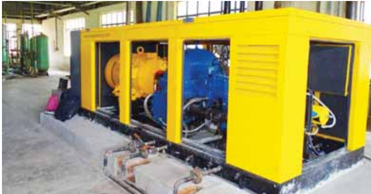
At Malanpur, we commissioned a 150 kW micro-turbine. This will help us convert pressure loss in steam lines into power, generate 100 kWh of power per annum.
