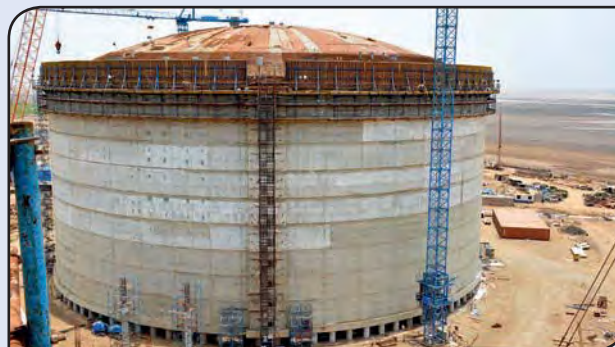
Expansion at Dahej Terminal
