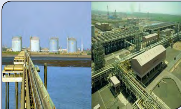
Expansion at Dahej Terminal
