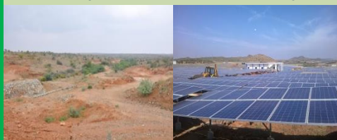
Ananthapuramu Solar Power Project
