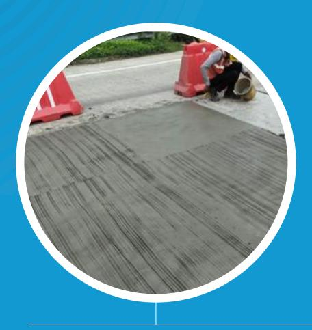
It is basically the plain concrete, or reinforced concrete slabs laid directly over the Dry Lean Concrete or a stabilized base course.
