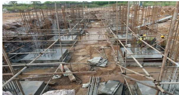
Captive power plant foundations
