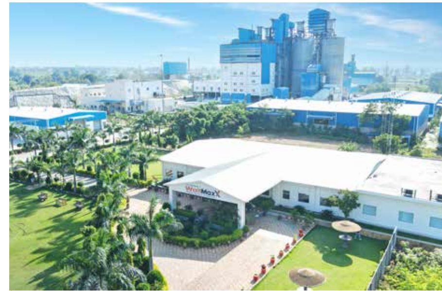
JK Cement Plant, Katni
