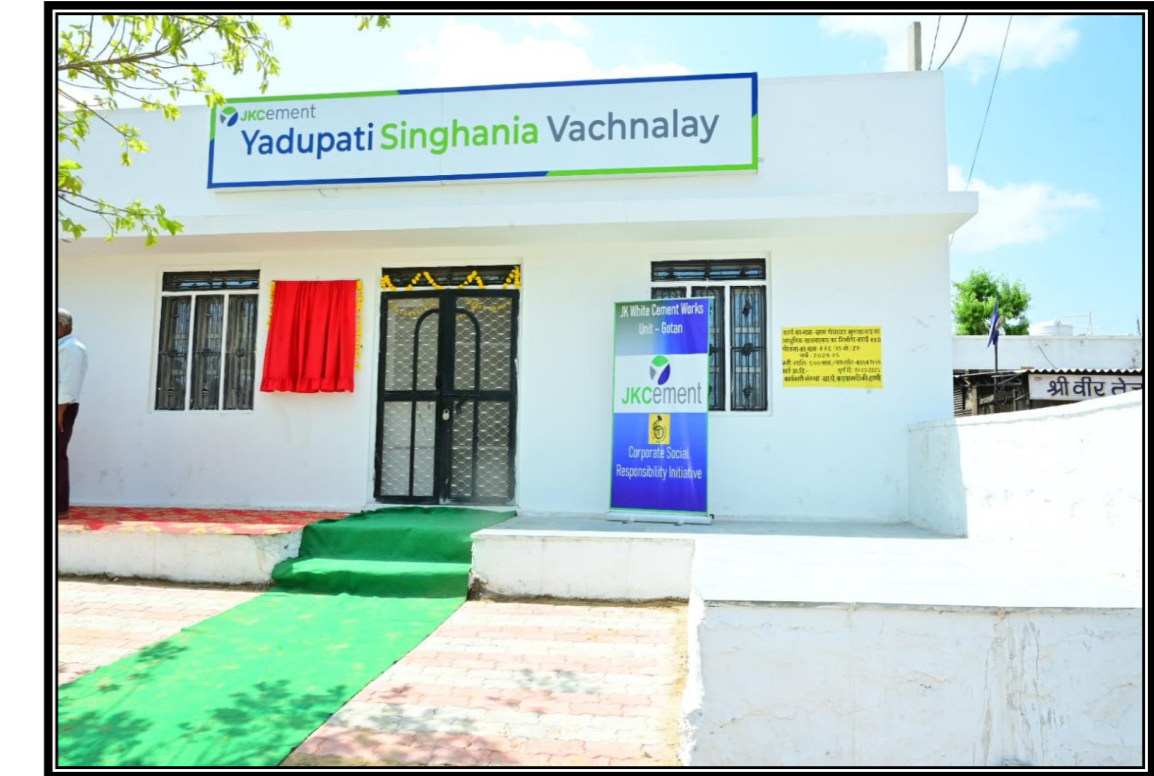
Construction of Vachnalay at Gotan
