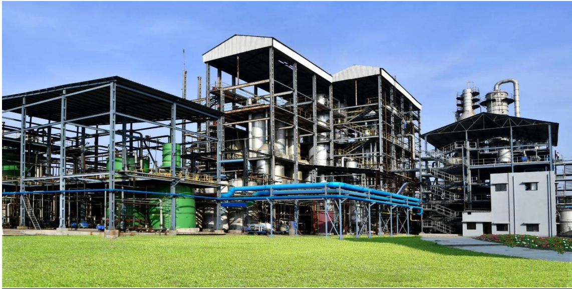
Cogeneration Plant at the Sameerwadi Manufacturing Facility
