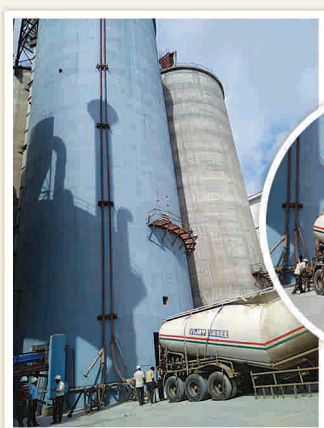
Converted Cement Silo to Fly Ash Silo
