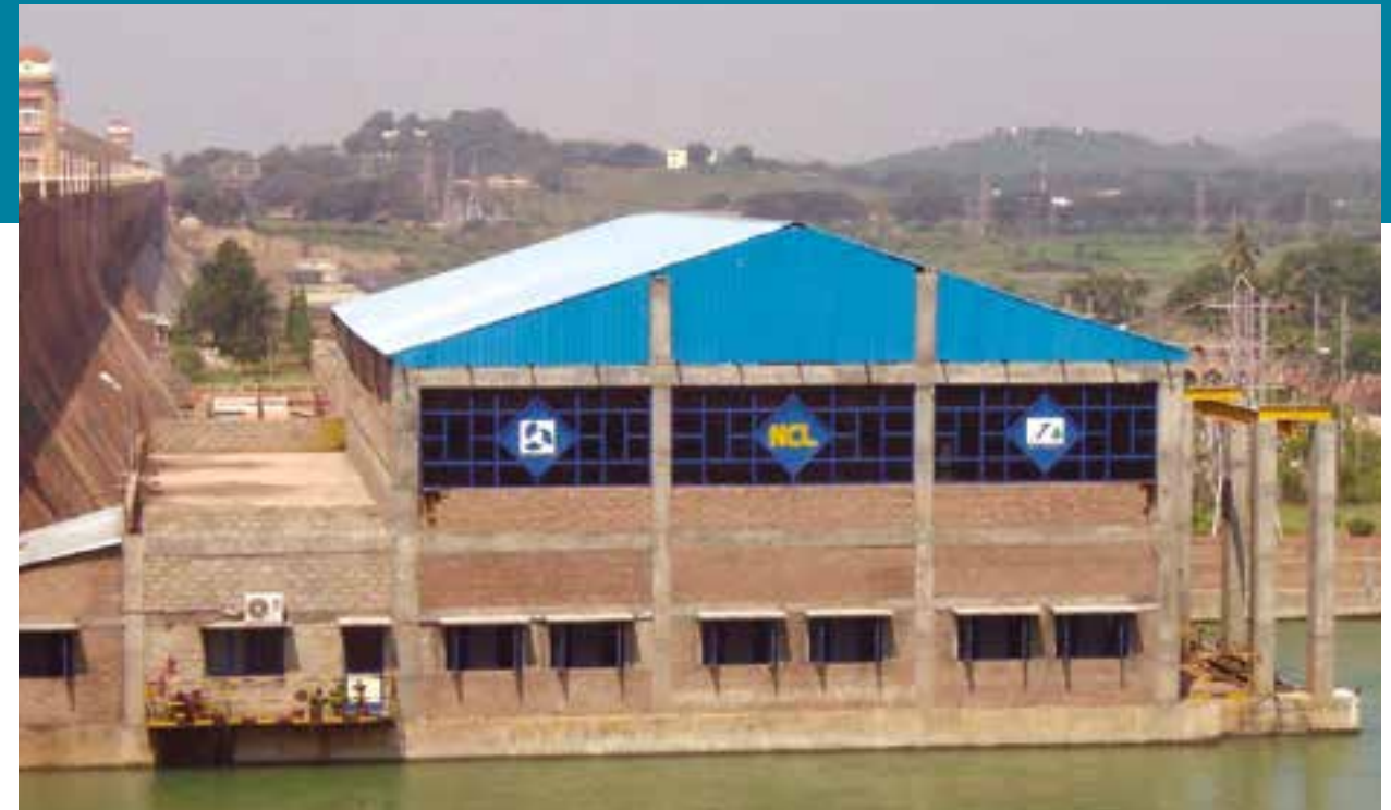
Hydel Power House at Tungabhadra Dam.
