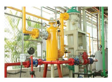
The heater less vapouriser installed at Wada Plant, which has replaced the 36kW electrical heater base vapouriser, has achieved energy saving of ₹5.1 lakhs/annum with a payback of 14 months
