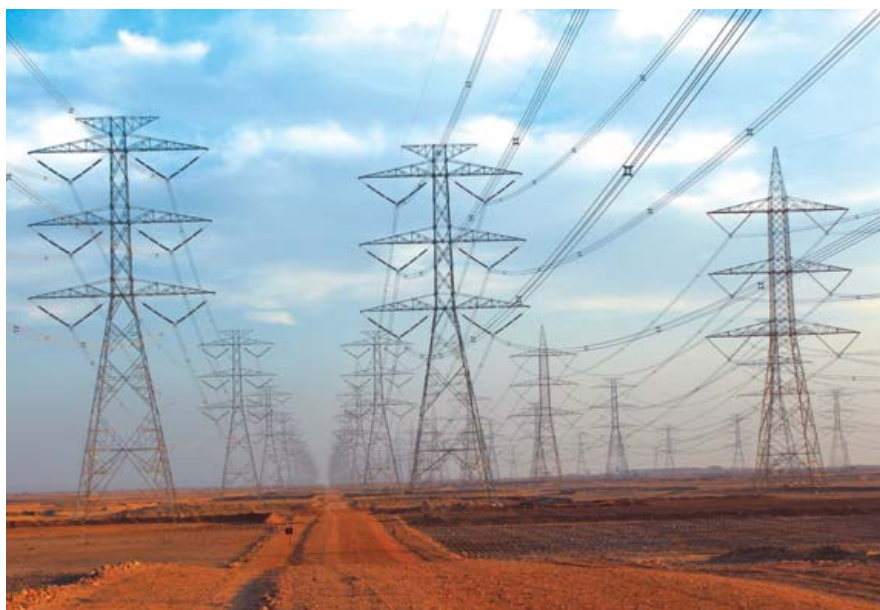
▶ 380 kV Double Circuit OHTL from Rabhigh IPP2 to Al Mashar Substation, Saudi Arabia
