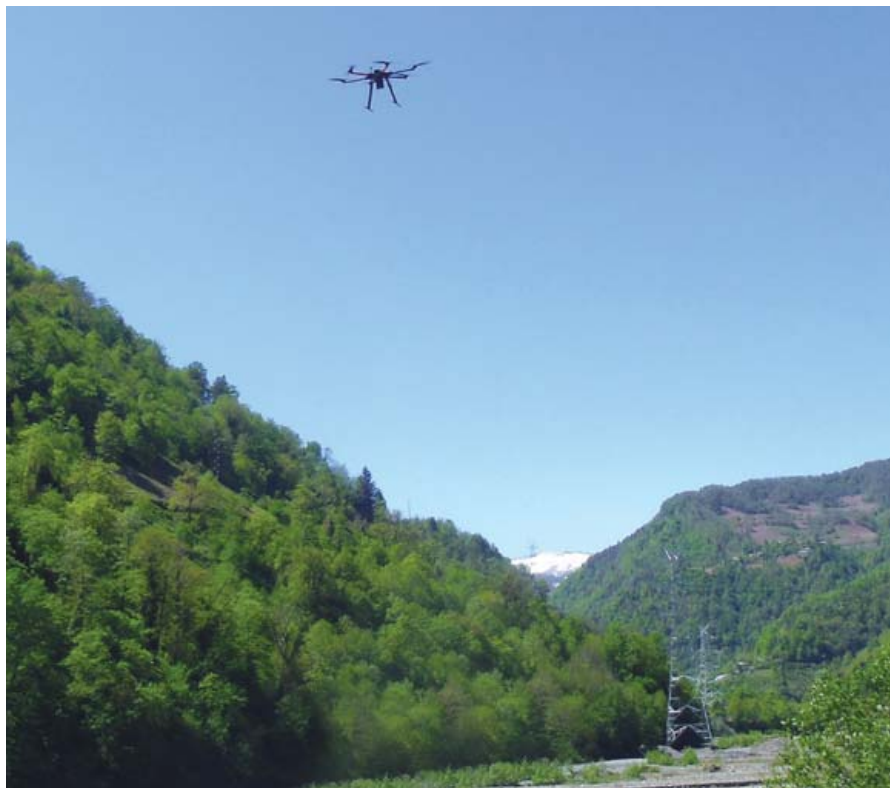
▶ Stringing Using Drone at Project Site in Georgia
