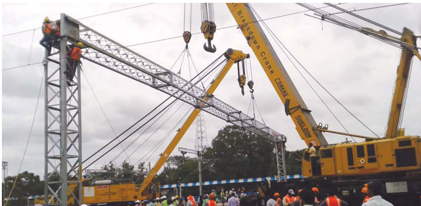
▶ 40 Meter Boom Erected for Railway Electrification Project at Daund Station, Pune, India
