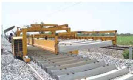
Sleeper laying in progress at Jhansi-Bhimsen Railway Project, Uttar Pradesh
