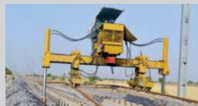
Track Laying Machine at Jhansi-Bhimsen Railway Project, Uttar Pradesh
