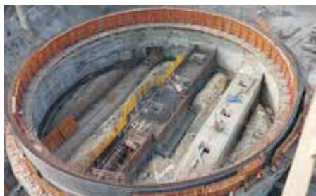
Specialised Climbing Formwork technology for construction of heavy silo structures
