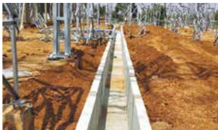
Precast Cable Trench for 220/66 kV Jagalur Extension project
