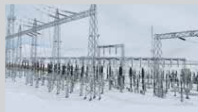
220 kV AIS Substation at Ghazni, Afghanistan
