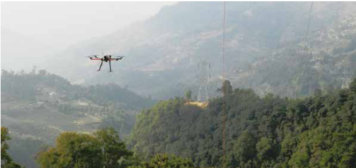
Stringing of power conductors using drone, Bhutan
