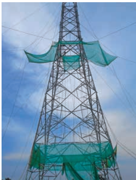
Safety net to minimise the impact of an unexpected fall
