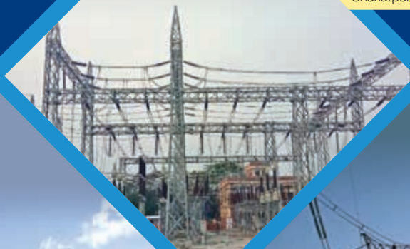
132 kV AIS Substation at Shariatpur, Bangladesh
