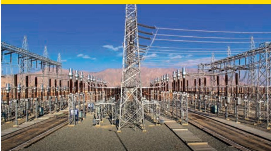
500/220 kV Dasht-e-Alwan AIS Substation at Pul-e-khumri, Afghanistan
