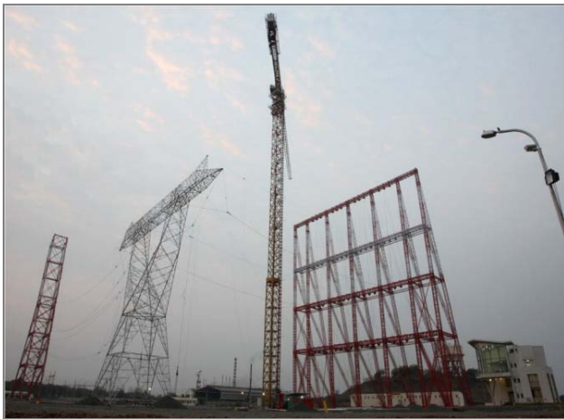
1200 kV Tower Testing Station at Nagpur
