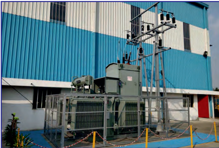
Skid mounted substation (SMS): SMS is an apt solution to Renewable power producers to meet expectations of short execution period at optimum cost
