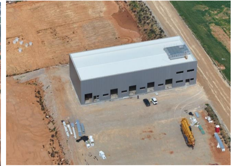
Maintenance Building External Wall Cladding
