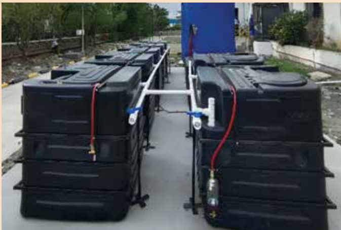
◀ BIOGAS PLANT GEARS- CHAKAN (70KG/DAY)
