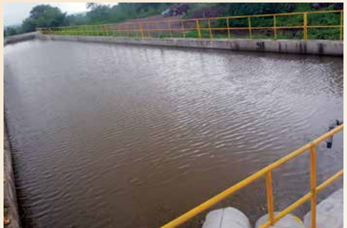
▶ RAINWATER COLLECTION CUM STORAGE AT COMPOSITE KANHE - 1800KL
