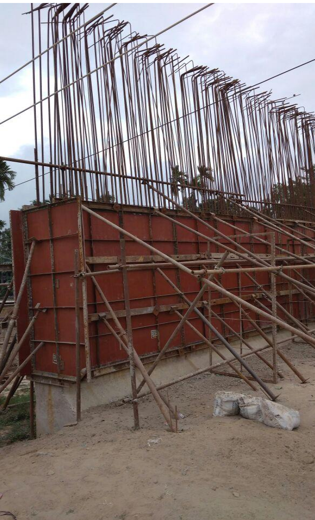
Vehicle Underpass at Moran Bypass of NH-37
