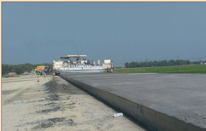
Cement Lining work in progress at Varanasi
