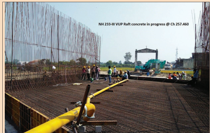
Raft concrete in progress at Varanasi
