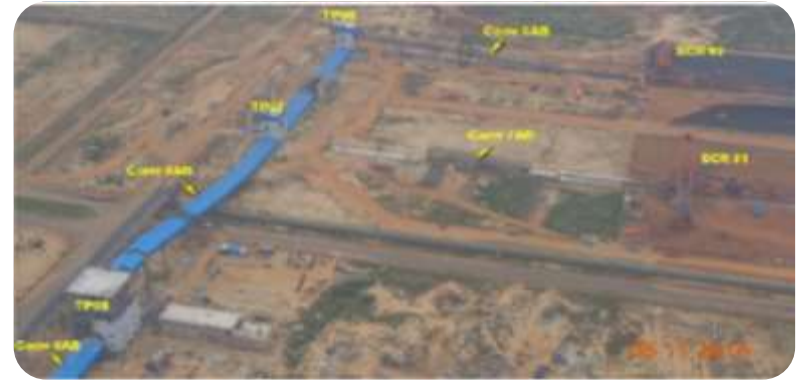
Internal coal handling plant
