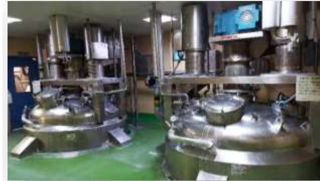
Main Mixing Tank
