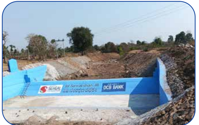
Constructed a check dam to conserve water, recharge groundwater, and support sustainable agricultural practices in the region, Medak, Telangana
