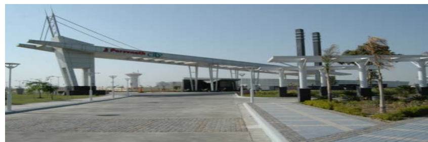
Parsvnath City, Sonepat, Actual Site Photograph
