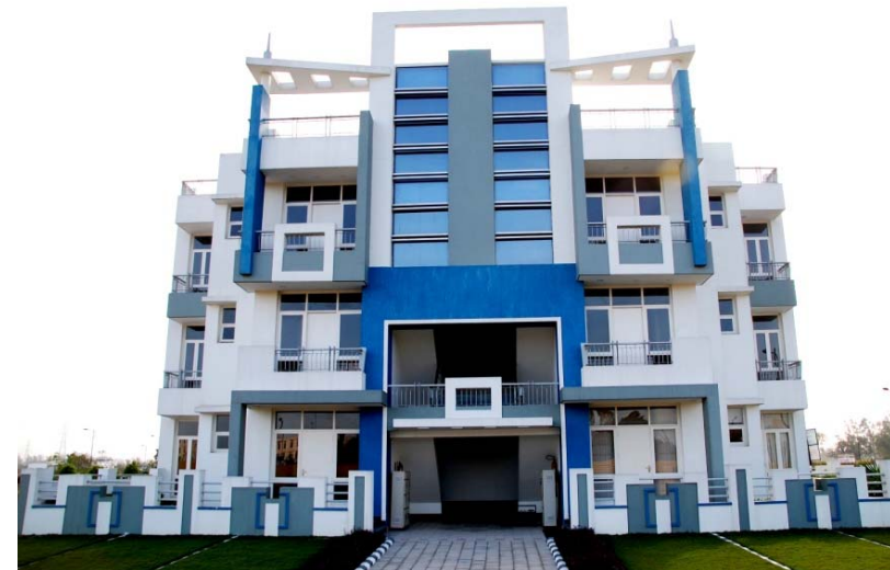
Parsvnath Royale Floors, Lucknow Actual Site Photograph
