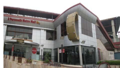
Parsvnath Metro Mall, Kashmere Gate
