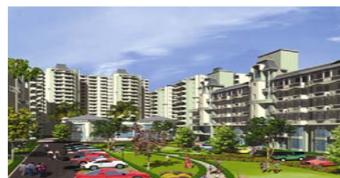
Parsvnath Green Ville, Gurgaon
