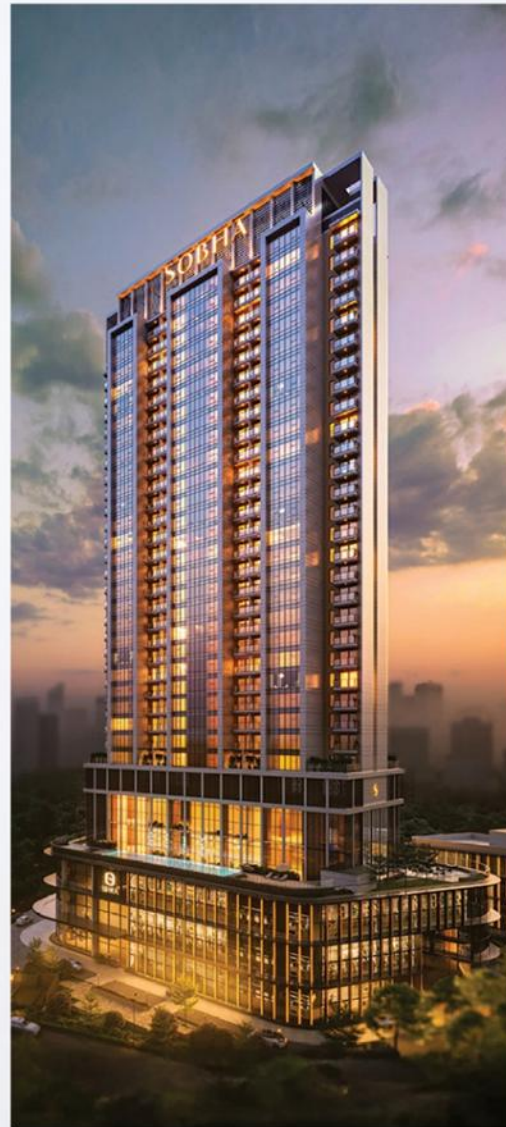
SOBHA Strada, Gurgaon
