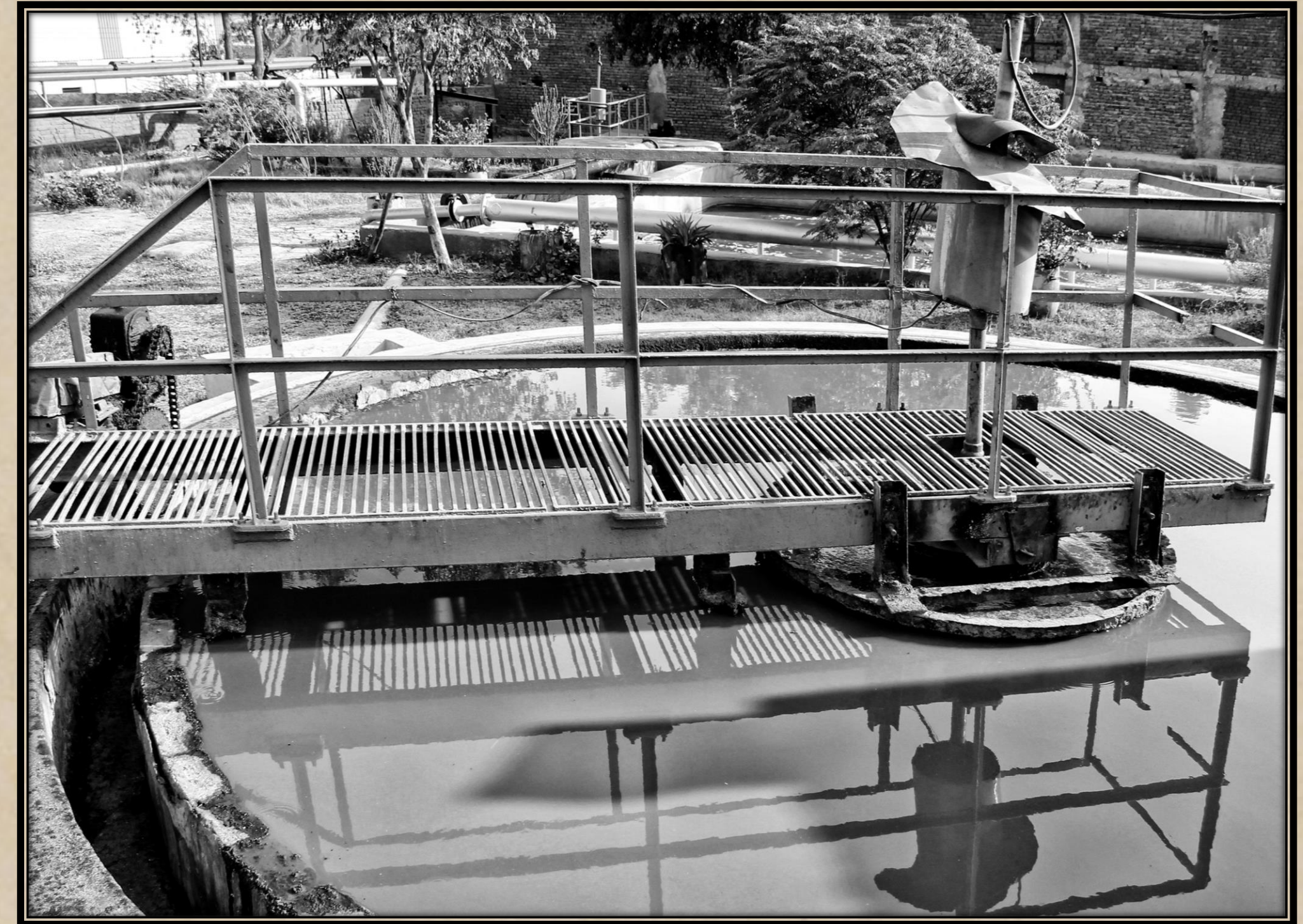
Effluent Treatment Plant - Our ETP is based on Activated Sludge process, adopted internationally all over world in Pulp & Paper Industry. It consists of Equalisation tank, Saveall, Primary Clarifier, Aeration and Secondary Clarifier.
