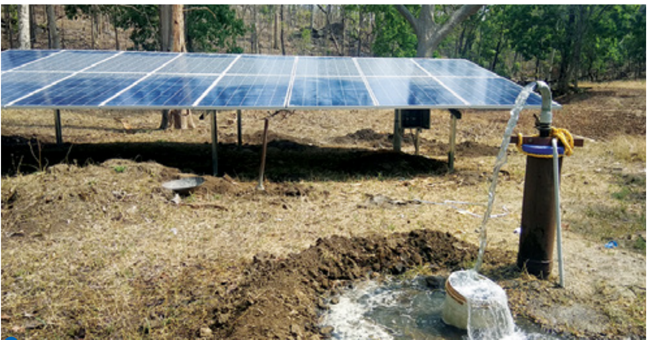
Installation of solar pumps in wildlife sanctuaries
