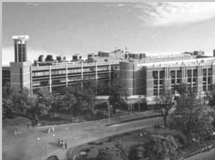
Fortis Hospital, Mohali
