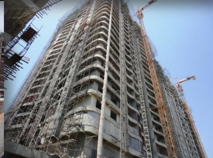
Metropolis- Near Completion Stage
