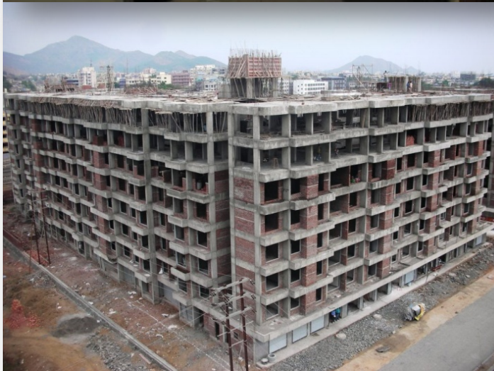
Residency Park Phase II- Near Completion Stage
