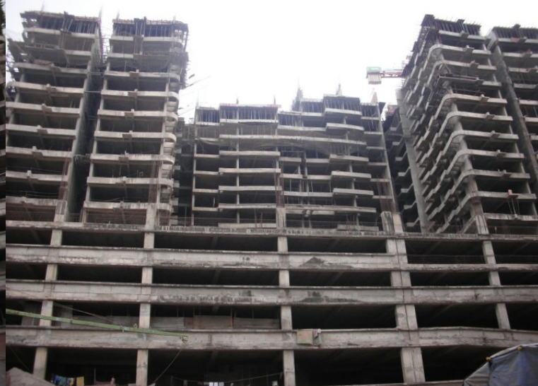
Majestic- Construction in Full Swing
