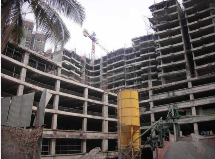
Majestic- Construction in Full Swing
