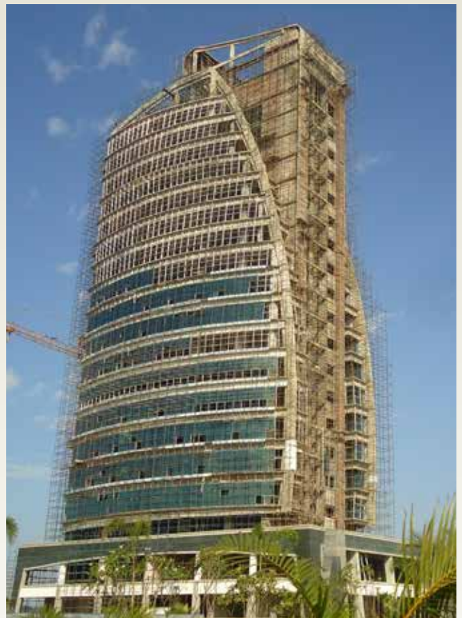
India Trade Tower, New Chandigarh
