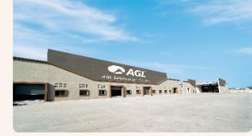
AGL Sanitaryware Plant
