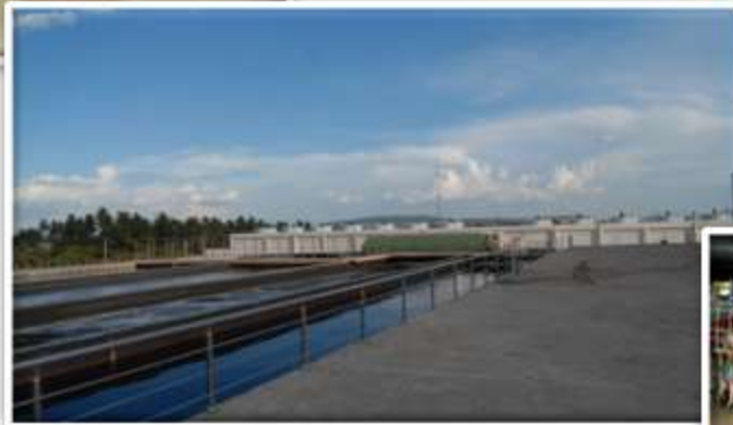
Effluent Treatment Plant, Sipcot
