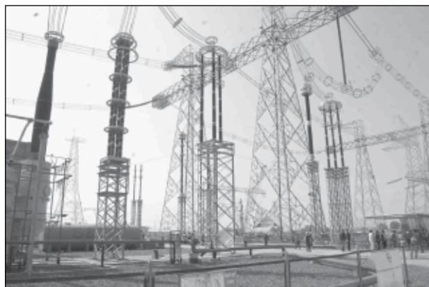
Fig: 1200kV (World's Highest Voltage level) bay at the National Test Station
