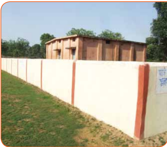
Boundary wall for a village school
