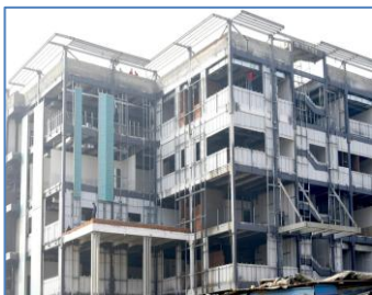
Commercial building, Delhi
