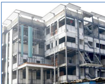
Commercial building, Delhi
