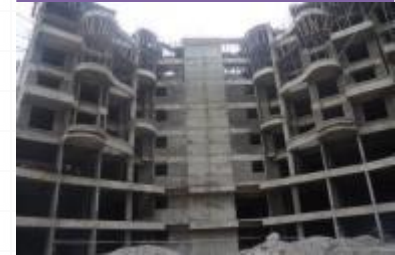
Site progress - June 2013
