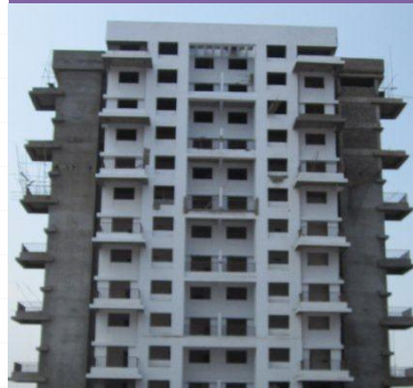
Site progress - April 2013
