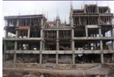
Site progress - June 2013
