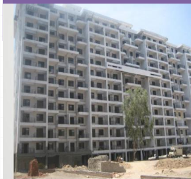
Flooring completed till 10th floor
