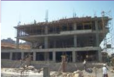
4th Slab in May 2013
