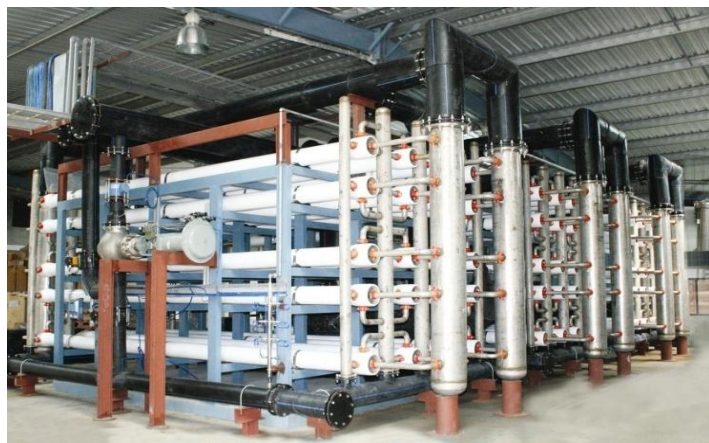
Effluent Recycling Plant – Tiruppur
