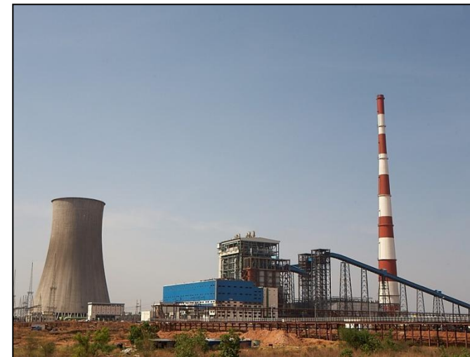
Kakatiya Thermal Power Station, Andhra Pradesh
