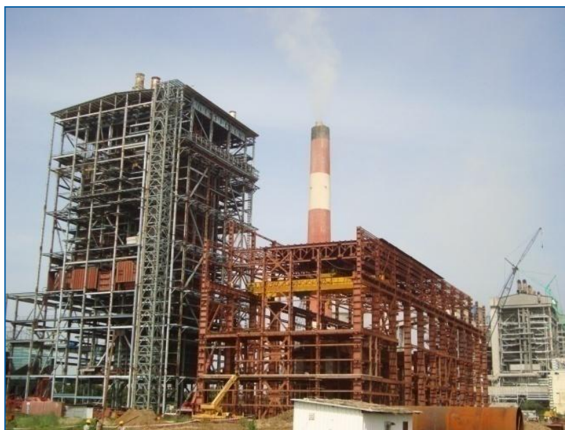
Kothagudem Thermal Power Station (Under Construction)
