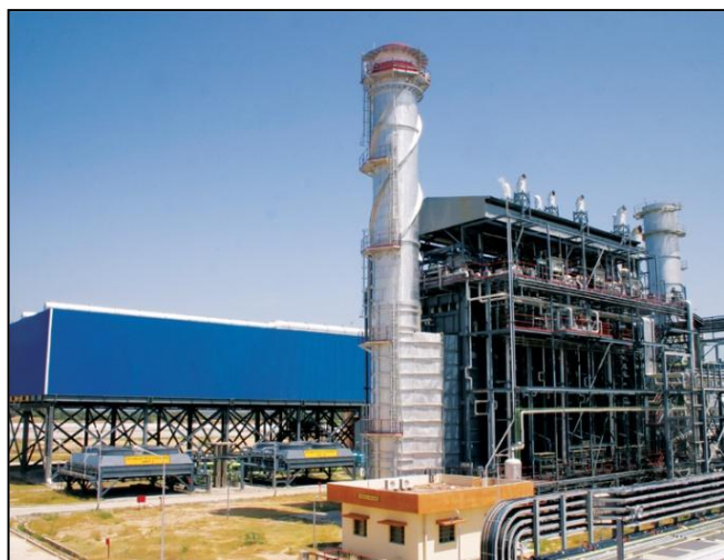
95 MW CCPP Valuthur (Phase I), Tamil Nadu
