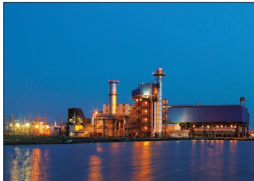
92.2 MW CCPP Valuthur (Phase II), Tamil Nadu
