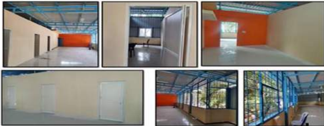
Renovation work at Subramanya Nagar Police Station
