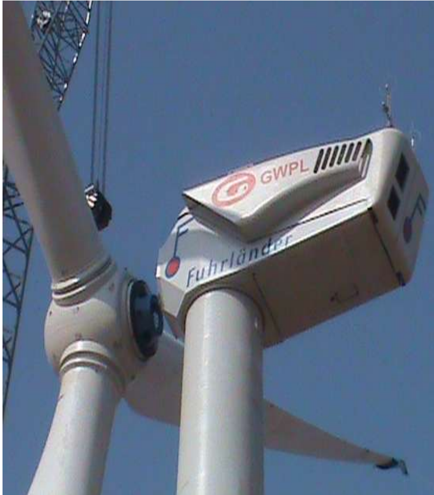
Rotor Hub erection in progress
